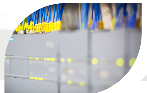
Control board with Siemens S7-1200 PLC
